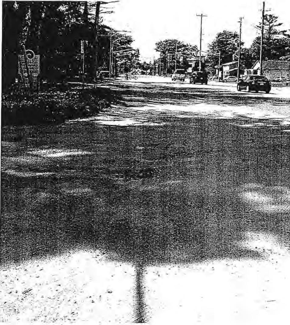
River Road West and Zoo Park. Sediment accumulation due to improper drainage.
