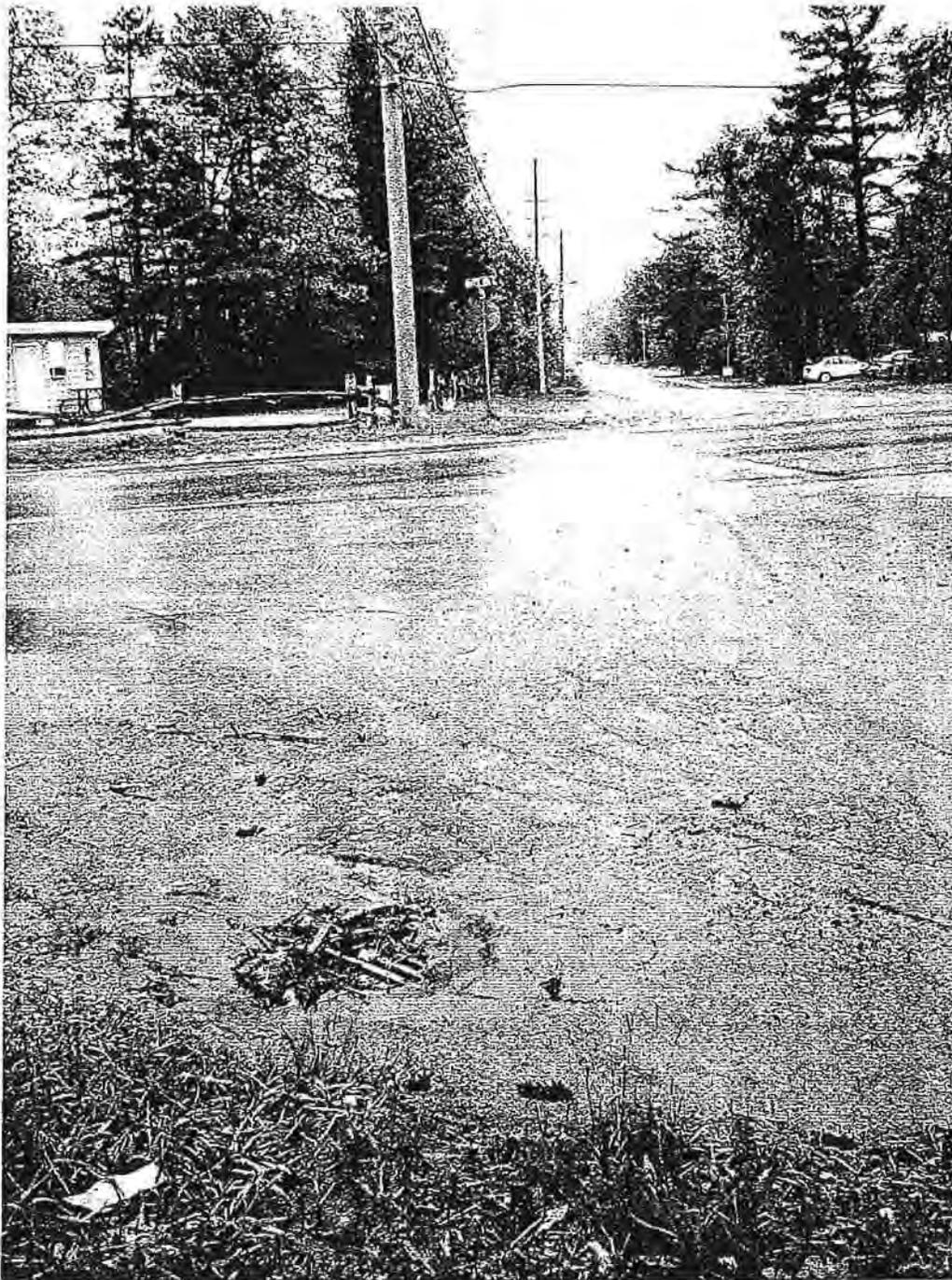
EXCESSIVE EROSION AND SEDIMENT ENTERING THE EXISTING STORM SEWER NETWORK.
