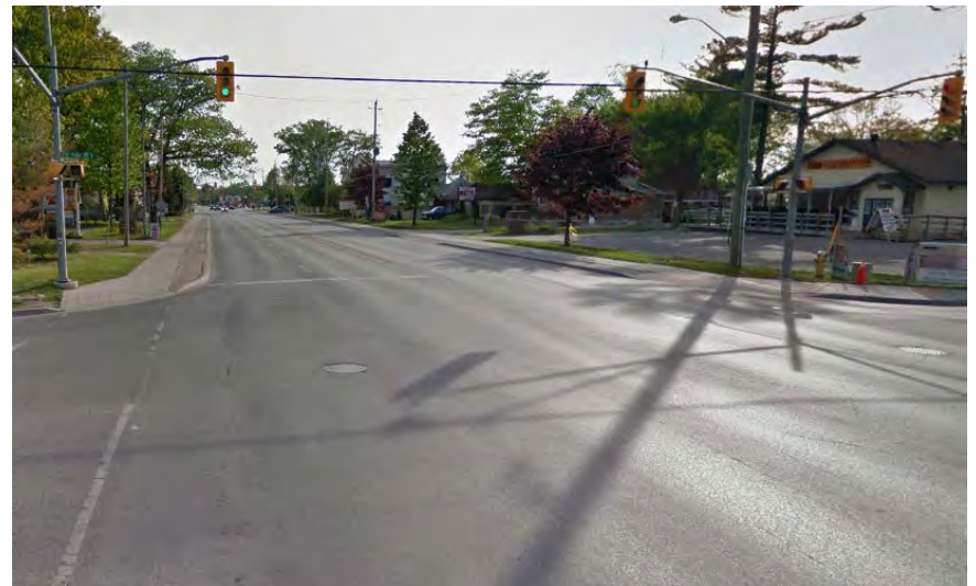
Looking west along River Road West from Zoo Park Road
