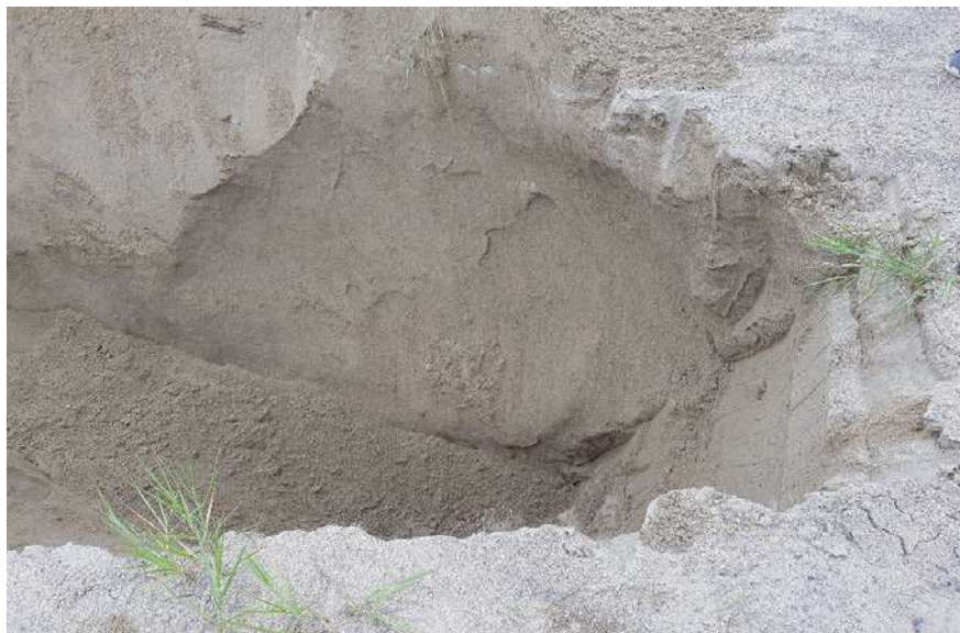
Photograph 2 - Test Pit 5 showing upper fill over native sand. Sidewall sloughing occurred within the fill.
