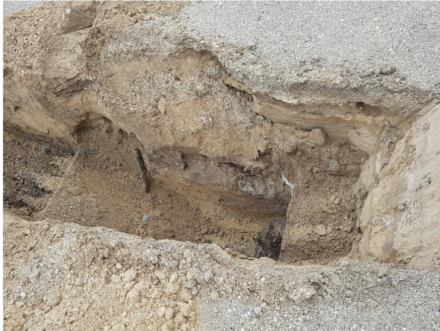
Photograph 2 - Test Pit 3 showing upper fill containing construction debris.
