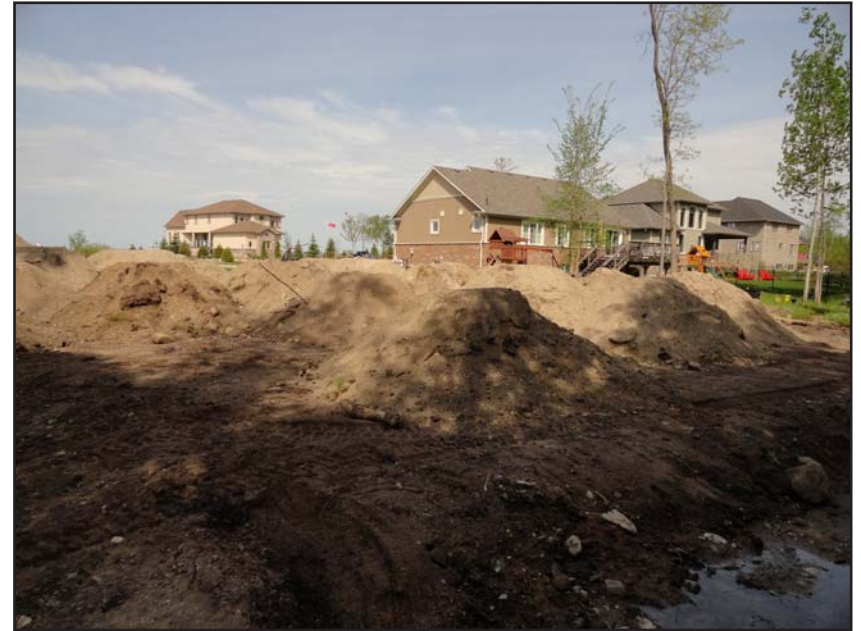
Photograph 2. As-built and on-going construction of single-family houses along Shore Lane, at north edge of property
