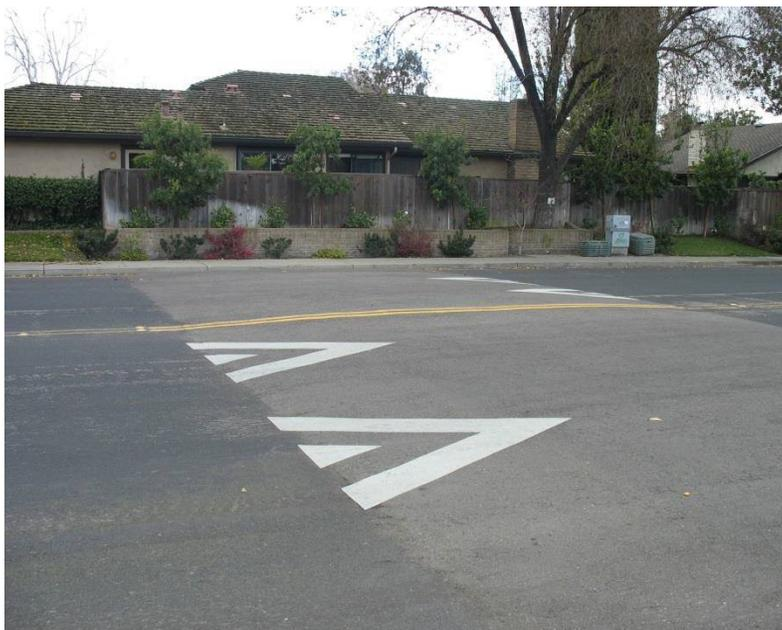
For an 85<sup>th</sup> percentile speed of approximately 40 km/h, the speed table should be 80 mm high and 6.5 metres long in the direction of travel (2 metre ramps at the ends and a 2.5 metre plateau which is typically long enough to accommodate the entire wheelbase of a passenger car).
