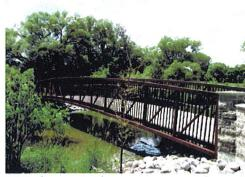
5.3 Pedestrian Bridges – 3.0metre wide steel prefabricated pedestrian bridges
