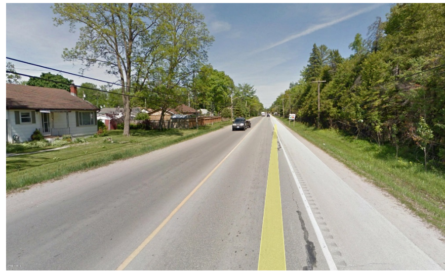
Looking east along Mosley St from 65 th St
