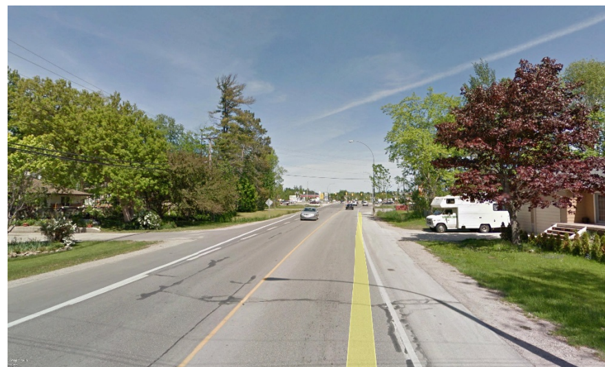
Looking east along Mosley St from 47 th St
