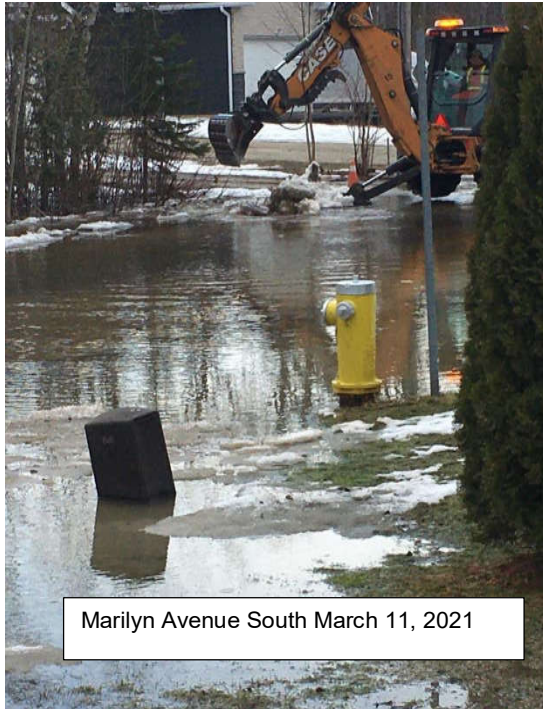
Marilyn Avenue South March 11, 2021. The road is underwater. The picture is taken from inside the garage at 16 Marilyn Ave S. Note the hydro substation.
